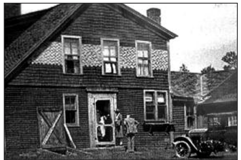
Note the bulkhead to the root cellar just to the left of the door. Also, note the unusual window layout.
