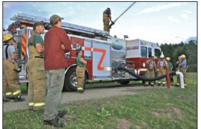
First test of the Dry Hydrant's ability to allow the North Haverhill Fire Department draw water from the lake in a more timely manner. "Success" Two more Dry Hydrants are scheduled for first of next year.
