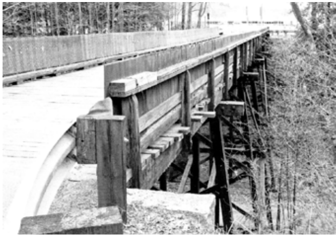
The Mill street bridge is scheduled for replacement in 2018.
