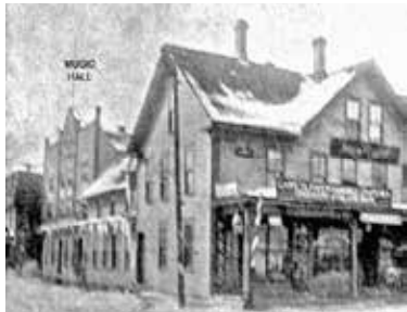
The new Music Hall quickly filled with businesses making the tiny Pleasant street commercially very active! Then on May 5th, 1901, disaster struck and both buildings burned to the ground!
