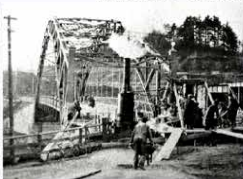
PAVING ABOUT FINISHED!
