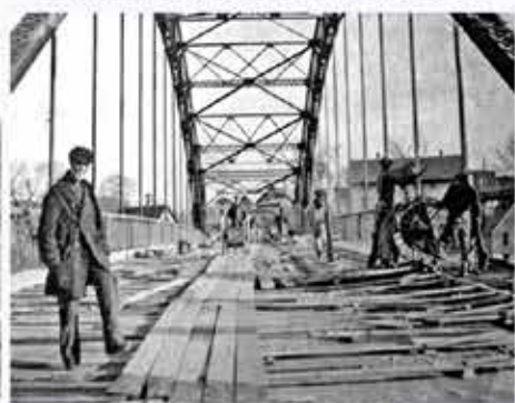
LAYING THE PLANKS
