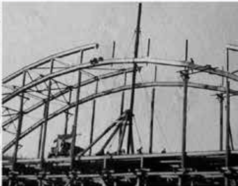
MEN ON TOP JOINING THE TWO SIDES
